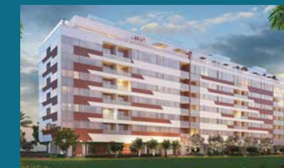
ÉLITON GONÇALVES By Real Engenharia SQNW 106 Bloco I - Noroeste
