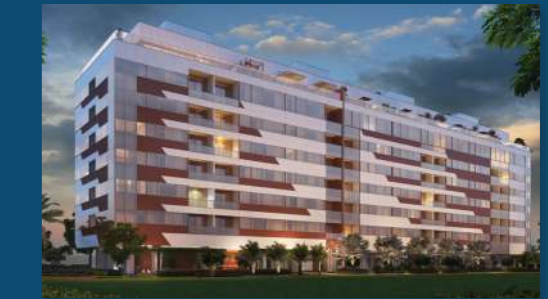
ÉLITON GONÇALVES By Real Engenharia SQNW 106 Bloco I - Noroeste
